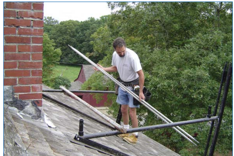
A mason restores the chimney at the John Greenleaf Whittier Birthplace.
